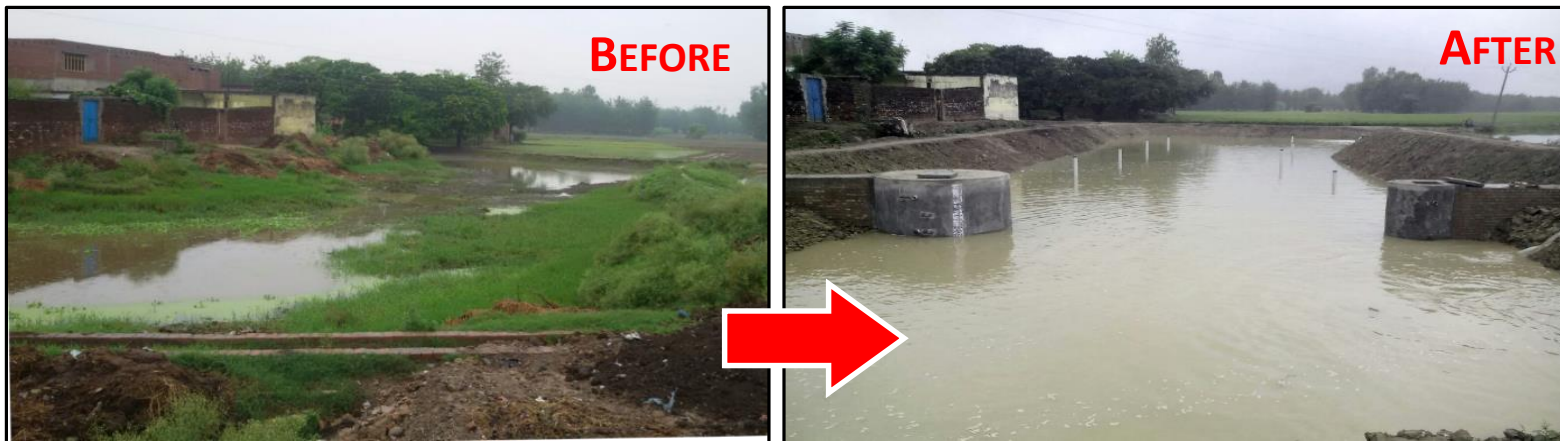
Community pond converted for UTFI in Jiwai Jadid village. The village is periodically flooded and groundwater levels have been falling, which impact on domestic water supplies and agricultural livelihoods.
